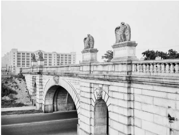
Colonial Road Bridge, Brooklyn August 1940
